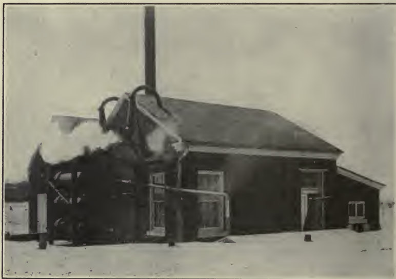
Fog signal at Cape Henry Light Station, Va.
