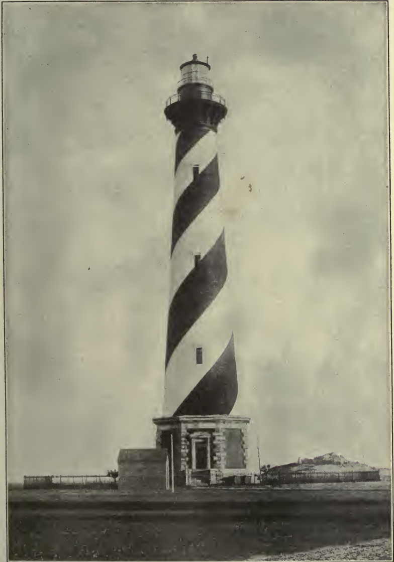
Cape Hatteras Light Station, N. C.
